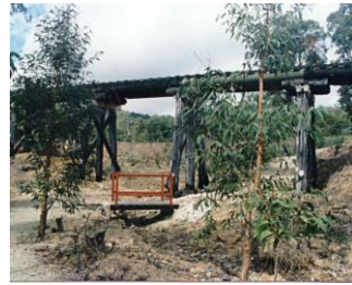
Prospectors Gully Rail Bridge
